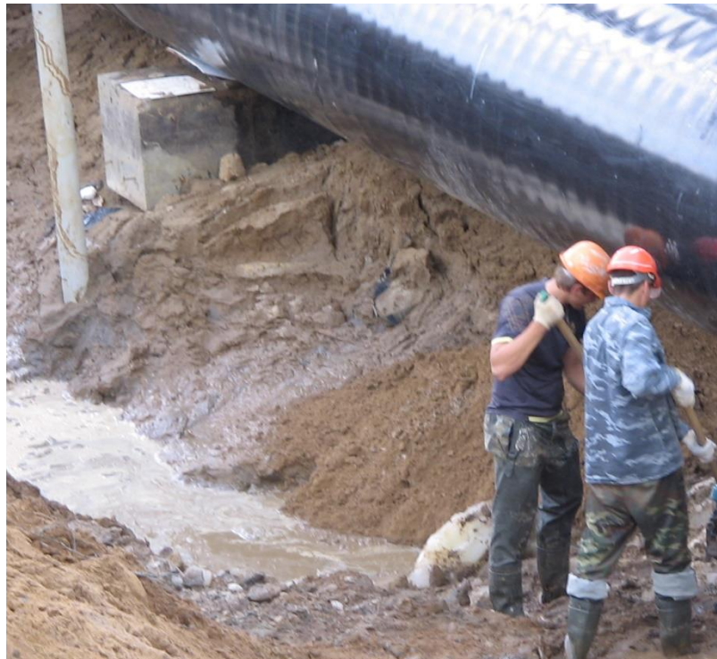
Figure 3 – July: ice underneath the exposed pipeline laid in winter is removed.
